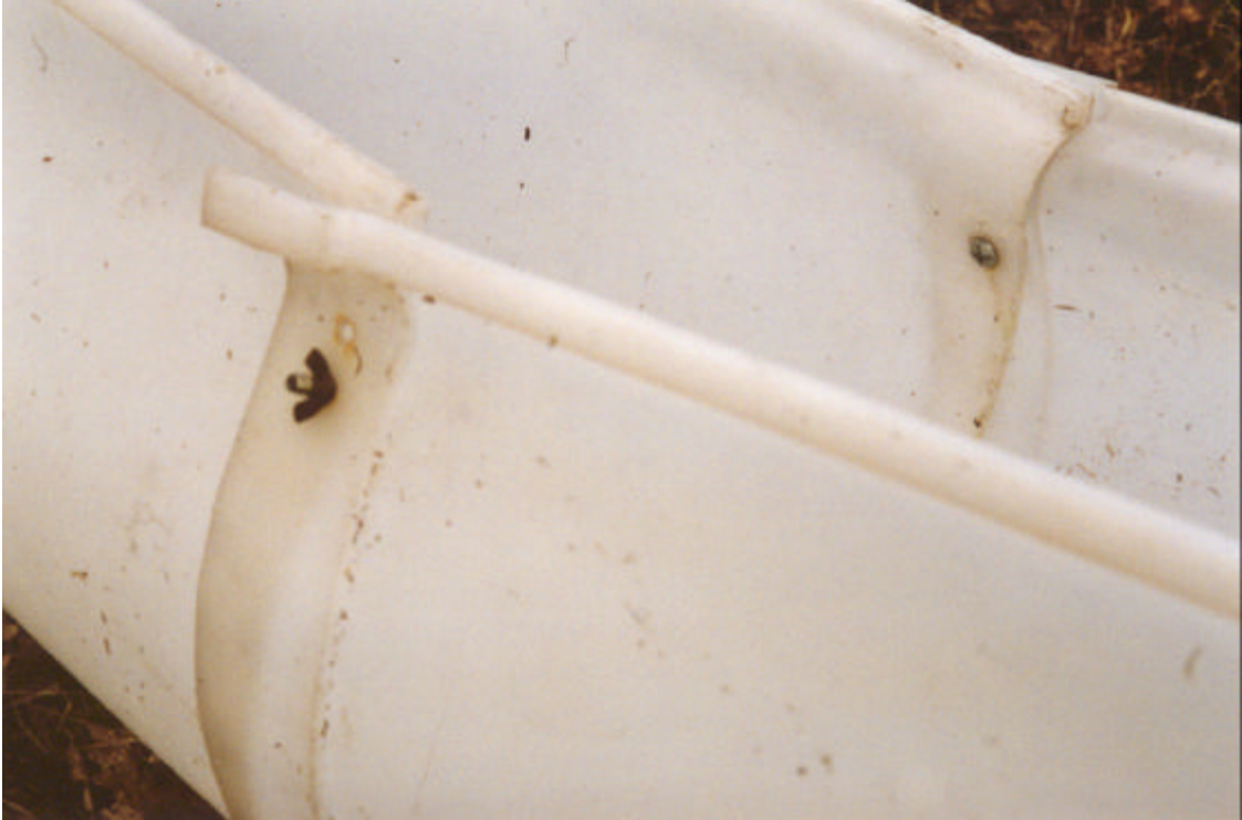
Plate 3 Wing Nut and Bolt Fixings
